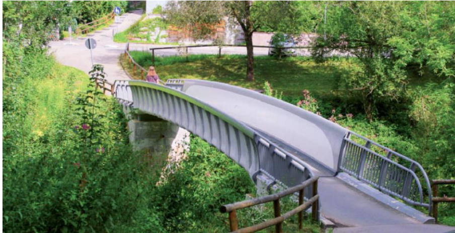
Figure 20- TRC bridge "Rottachsteg" in Kempten [96].
