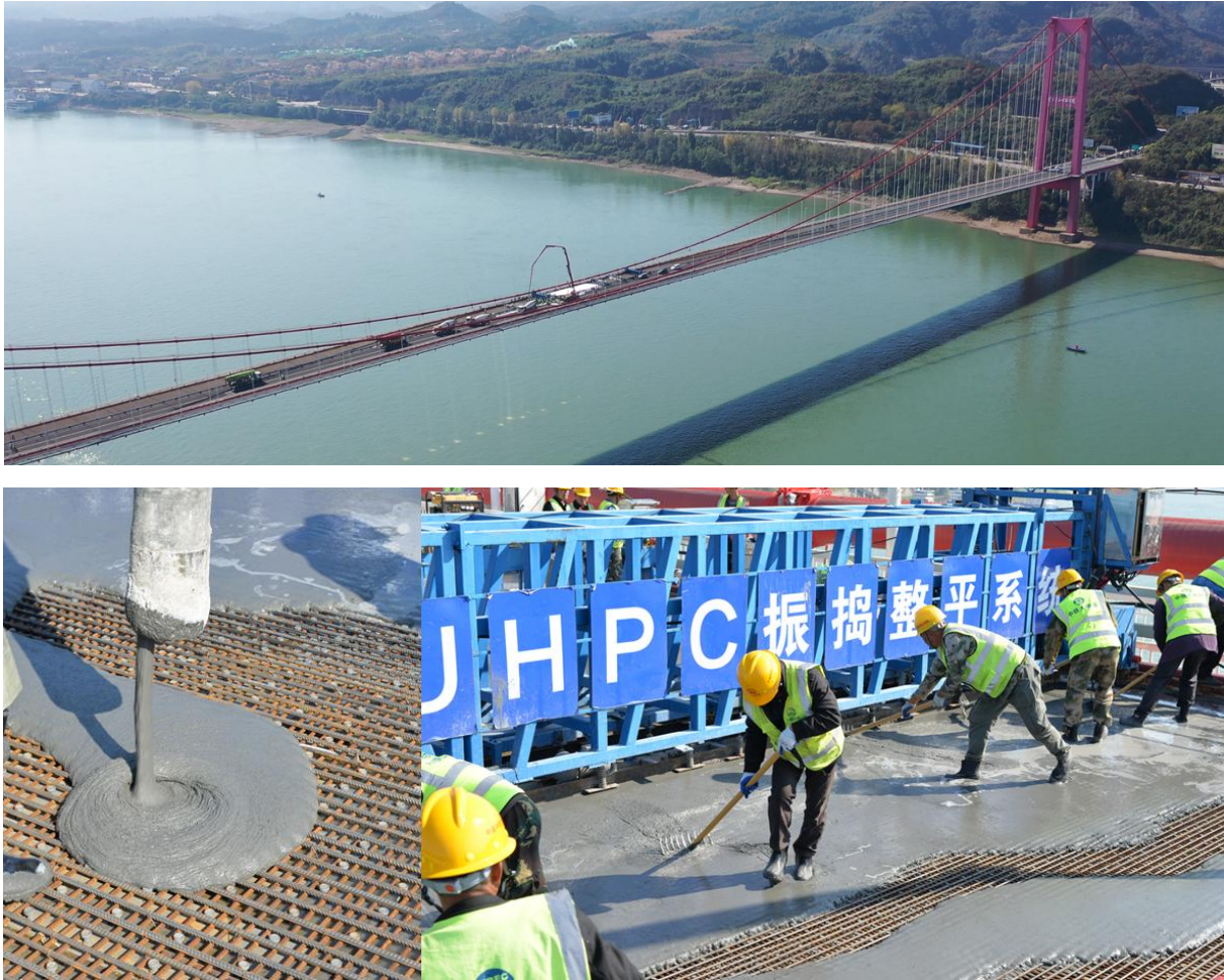
Figure 11 Orthotropic steel deck (OSD) strengthening using UHPFRC: Examples in China
