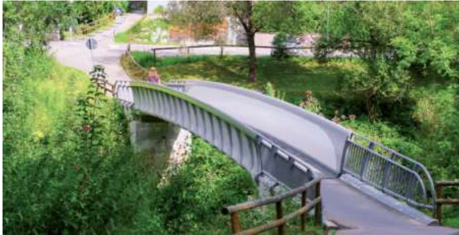
Figure 20- TRC bridge "Rottachsteg" in Kempten [96].
