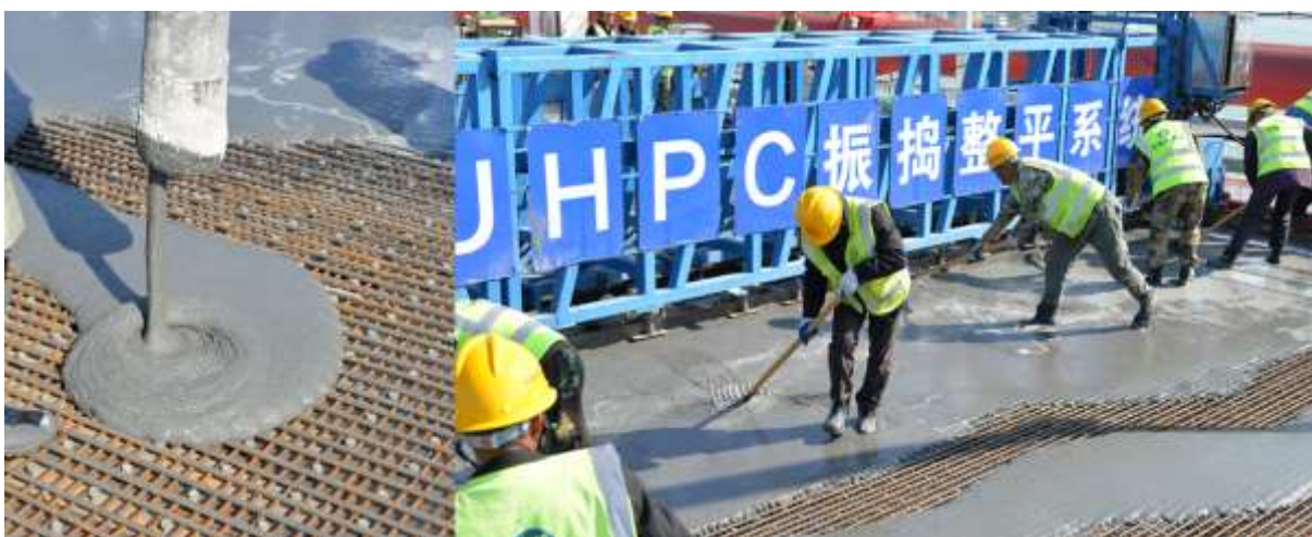
Figure 11 Orthotropic steel deck (OSD) strengthening using UHPFRC: Examples in China
