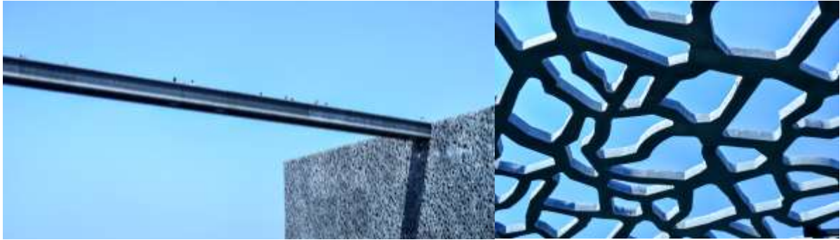
Figure 12 New structures using UHPFRC: (a) Le Bouveret footbridge in Switzerland; (b) Republic road bridge in Montpellier, France; (c) footbridge and facade elements in UHPFRC of the MUCEM building in Marseille, France
