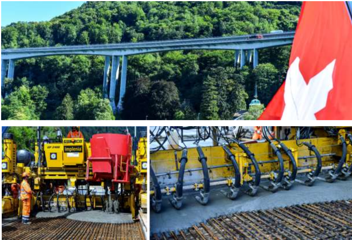
Figure 10 Reinforced concrete bridge deck strengthening using UHPFRC: Examples in Switzerland
