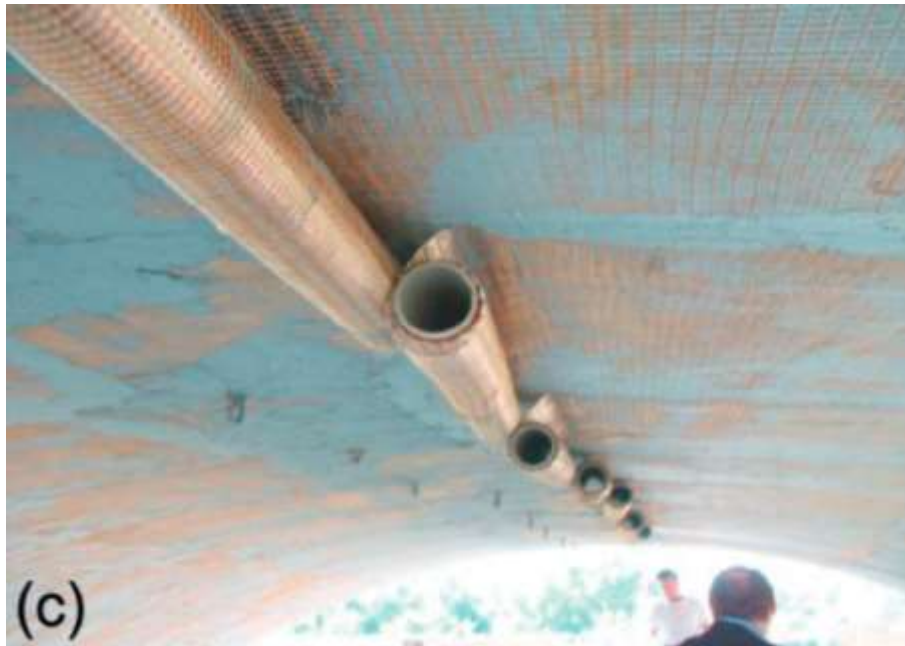
Figure 18- Strengthening of a bridge on the Rome-Formia-Naples railway [58].
