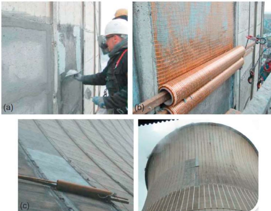
Figure 19 Procedure of strengthening application of a cooling tower in Germany [58].
